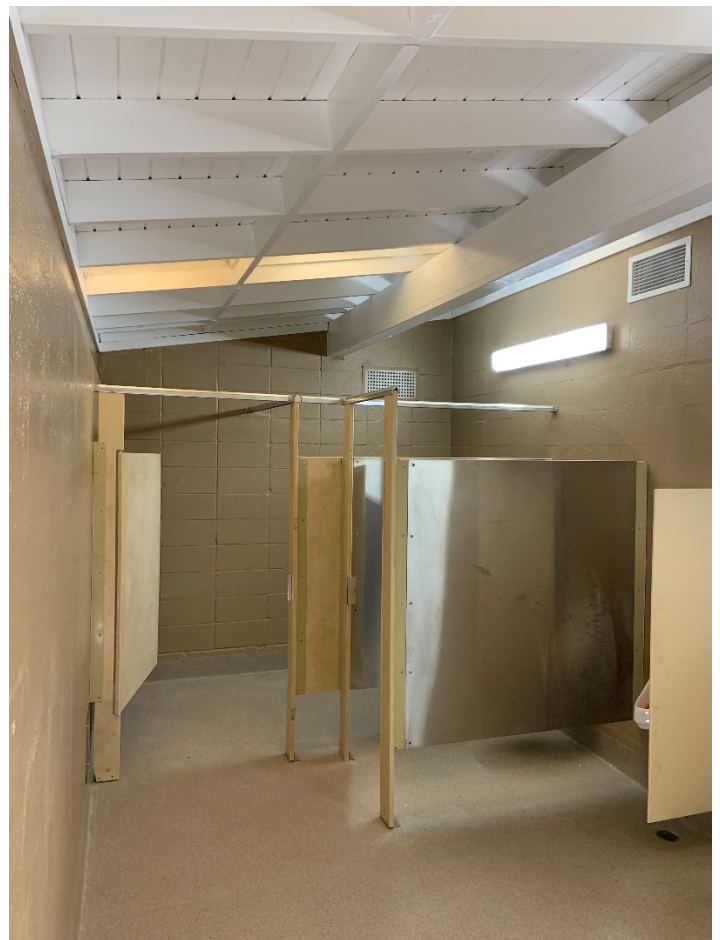
Figure 1- Van Duzer Restroom Remodel
