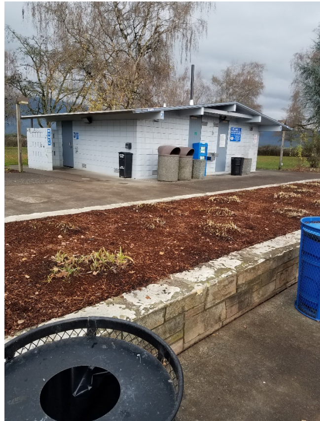
Existing Restroom Facility at Oak Grove Rest Area
